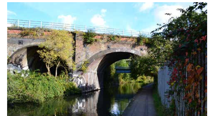
Railway Bridge No 8B, Grand Union Canal
