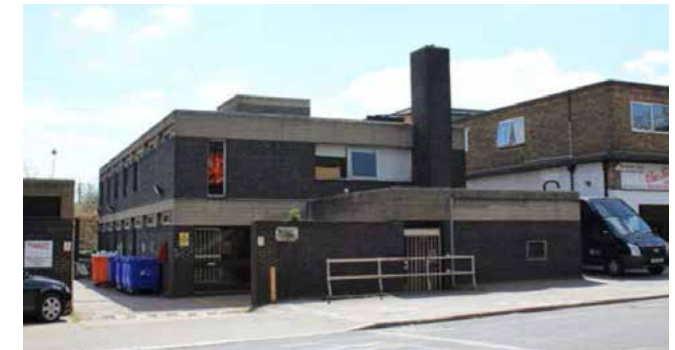
Former Willesden Junction Maintenance Depot, Old Oak Lane
